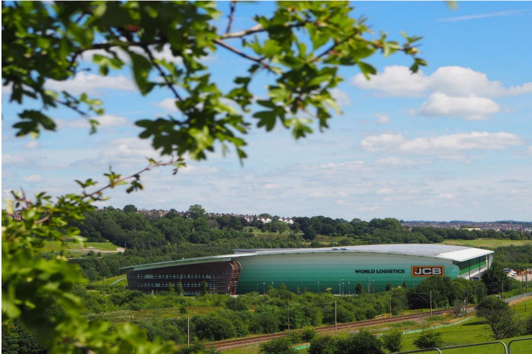
JCB World Logistics Centre on Chatterley Valley - the innovative building has a BREEAM 'excellent' rating.
